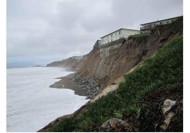
Coastal Erosion Mitigation
